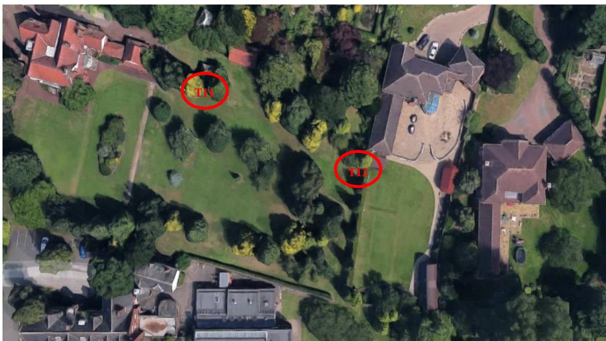
Figure 6. Tunnels 11 and 12 at Inglewood, Oadby Student Village
