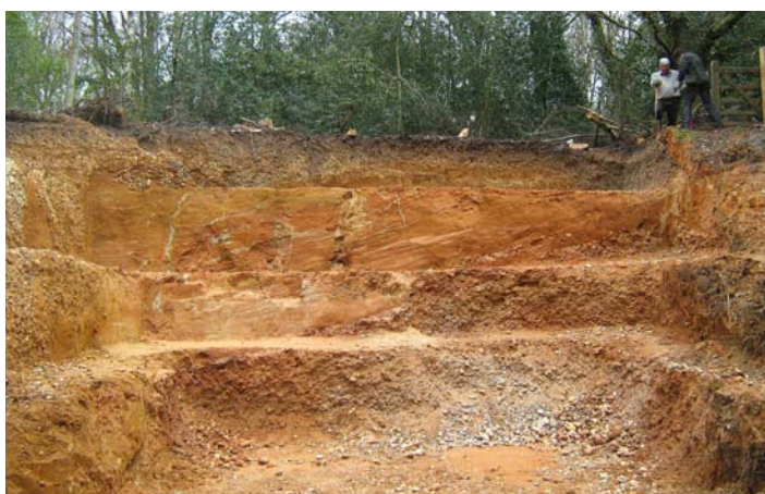
The site at Little Heath. Photo John Catt.
