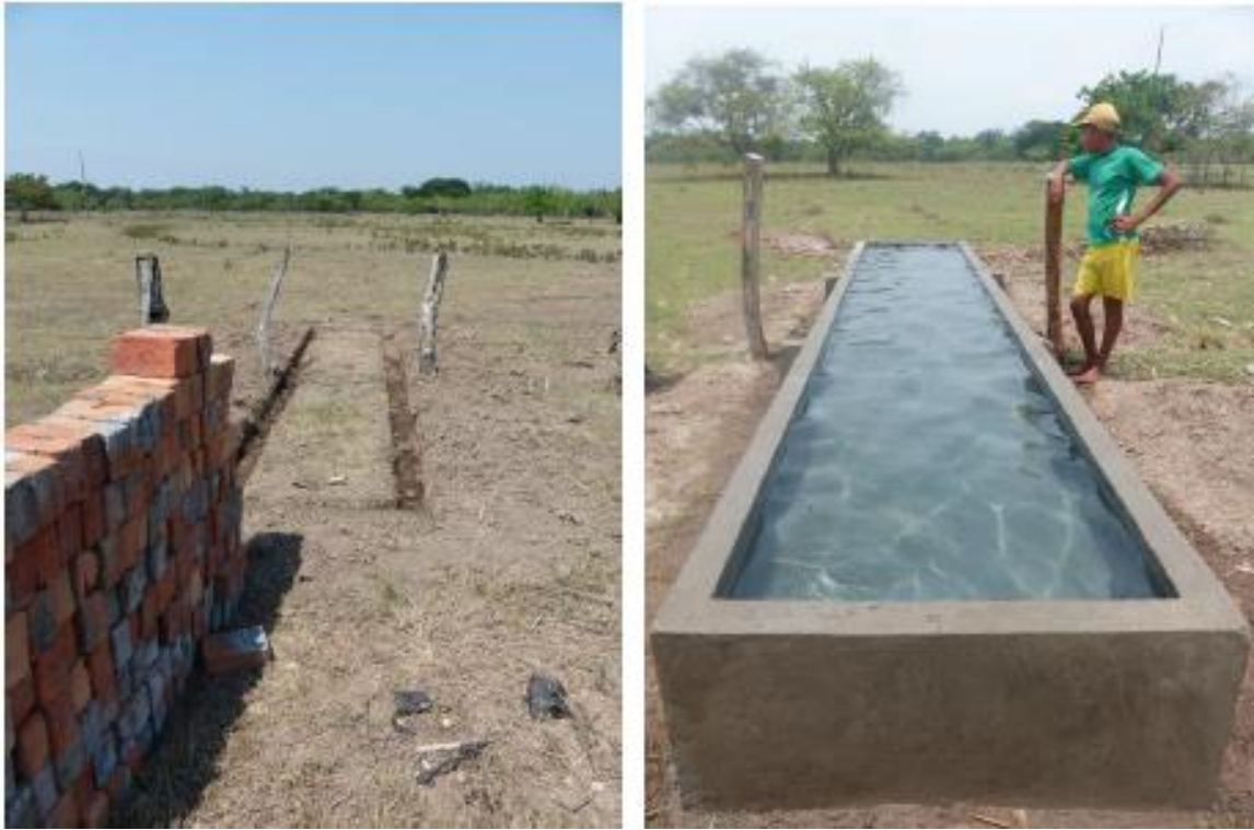
Figure 4. Livestock watering system to replace the water that cattle was drinking from the stream.
